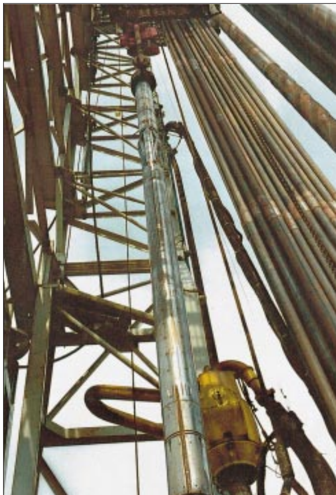
For simultaneous drilling and reaming operations, Cambridge Drilling Automation's automated guidance system has achieved impressive results including a single 7,100 ft run for Amoco Corp. The tool configuration includes a 12¼-in. hole size followed by a 14-in. reamer (Fig. 3).
